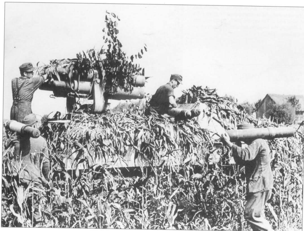
Crewmen prepare a Panzerwerfer for a fire mission while concealed in a crop field. This version was designated Sd.Kfz. 4/1 and consisted of an armored Maultier body with a ten-shot 15cm Nebelwerfer-Zehnling 42 launcher mounted on the roof. The tubes could traverse 360-degrees and fire ten 15cm high-explosive or smoke rockets out to about 6900 meters. Ten additional rockets were stored internally.
