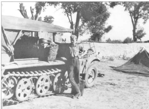
This Sd.Kfz. 10 has a camouflage scheme consisting of a lighter color brushed on in short strokes over its base paint, as can be seen below the radiator grill. Note the empty Notek lamp mount and the unusually uncluttered appearance of the tractor. The gun is a 7.5cm PaK 40, which can be identified by the shield configuration as well as the wheels with eight spokes. Modelers should note that the PaK has covers on the breech and the muzzle brake.
