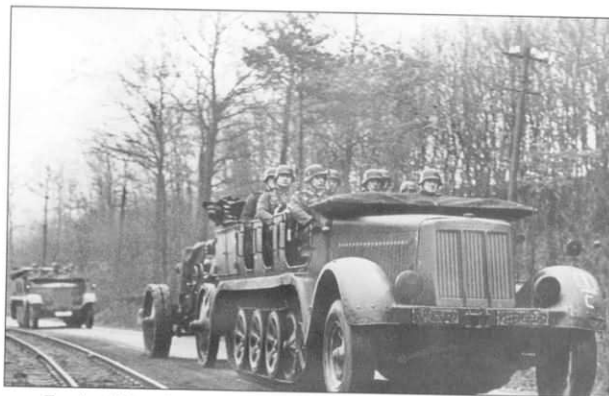
Tractor "C" pulls its gun alongside a railway line. As the vehicle is relatively pristine and the crew rather clean-looking, it would appear that they are on a training mission. The lack of a Notek black-out driving lamp would place this vehicle early in the war, or what is more likely, pre-war. Note also the rod-style grab handles along its sides, between the rows of seats.
