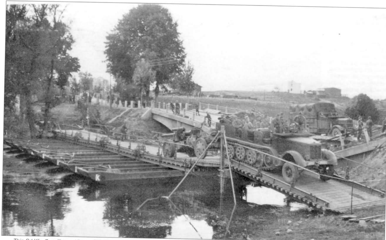
This Sd.Kfz. 7, pulling a 15cm s.FH 18, crosses a river on a pontoon bridge previously constructed by members of a Pioneer Brukenkolonne (Engineer Bridging Column). Next to it, the original civilian bridge that was partially destroyed is being used for lighter vehicular traffic, in this case what appears to be a Henschel 33D1 truck. The tractor has no Notek lamp mounted, while the howitzer has the pierced, dish-style wheels on the carriage and limber.
