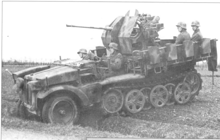
This familiar photo shows a beautifully camouflage-painted Sd.Kfz. 10/5 mounting a shielded 2cm Flak 38. Note that the crewmen's helmets are also painted to match the vehicle, which itself is in a three-tone scheme of Dunkelgelb RAL 7028 base, with a blotch pattern of Rotbraun RAL 8017 and Olivgrün RAL 6003. This vehicle is fitted with second pattern road wheels, enclosed rifle racks and Notek black-out driving lamp.
