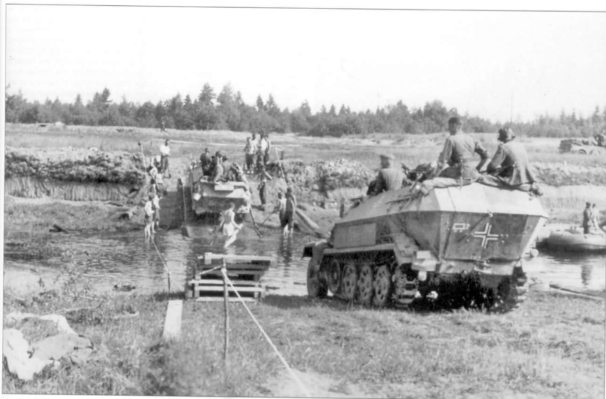
A Sd.Kfz. 251/1 Ausf. B prepares to cross a small stream with the help of Pioneers. Note the primary external difference from the previous Ausf. A: only one view port, instead of three, on the superstructure armor sides. This vehicle has a Notek tail-lamp fitted which would date it as post-1940. Note the Tac marking for a motorized rifle company and the lower-than-usual position of the Balkenkreuz national insignia.
