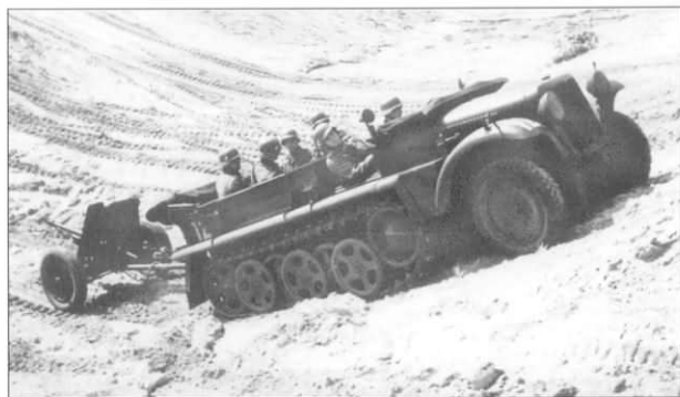
A Sd.Kfz. 10 pulls a 3.7cm PaK 36 up a rather steep embankment. Note the large white number "12" on the front fenders and the rear of the superstructure. The windshield has a canvas cover to eliminate reflections, while the road wheels are of the "first" pattern. There is no Notek lamp fitted. The PaK sports a small cap for the muzzle and there is a brake line that can be seen hanging down below the tubular trail arms.
