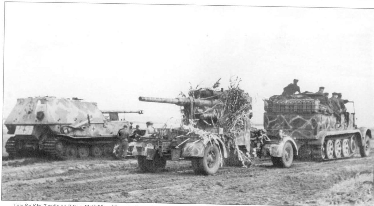
This Sd.Kfz. 7 pulls an 8.8cm Flak 36 or 37 past a Panzerjäger Tiger (P) "Ferdinand". The Flak gun features the later R.A. 9 multi-section gun tube and is mounted on the Sd.Ah. 203 limber system. Both tractor and gun are painted in a fairly complex camouflage scheme consisting of a "web" pattern created by spraying a lighter color over the darker base color.
