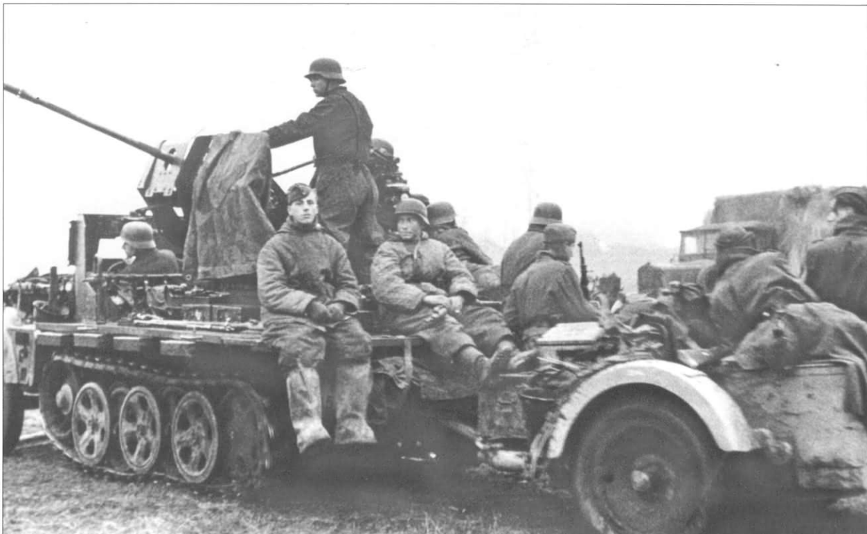
Armed with a shielded 2cm FlaK 30, this partially armored Sd.Kfz. 10/4 and its Sd.Ah. 51 trailer, along with a weary crew, take their rest. Note the spare magazine containers on the drop-sides as well as ammunition boxes on the platform below the gun mount. The FlaK 30 had a practical rate of fire of 120 rounds-per-minute, with a maximum horizontal range of 4800 meters. The gun's effective ceiling was 2000 meters, due to the fact that tracer rounds burned out at that distance.
