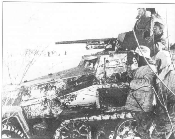
This Sd.Kfz. 251/10 Ausf. B sports a very scruffy and worn winter white camouflage, as well as the abbreviated sandwich-style gun-shield for the PaK 36.
