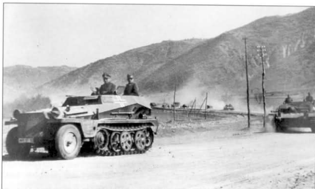
Captured Red Army troops take their rest in the lee of a hill, guarded by a Sd.Kfz. 253. Just visible on the forward portion of the '253's roof is the rotating cupola, which mounted a S.F. scissors periscope. The crewman is standing in the square opening of the rear hatch.
