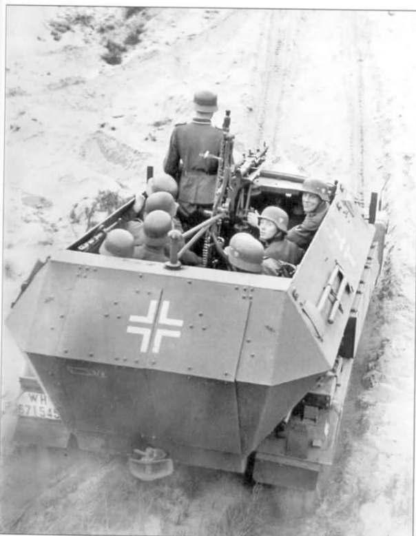
A Sd.Kfz. 251/1 Ausf. B prepares to cross a small stream with the help of Pioneers. Note the primary external difference from the previous Ausf. A: only one view port, instead of three, on the superstructure armor sides. This vehicle has a Notek tail-lamp fitted which would date it as post-1940. Note the Tac marking for a motorized rifle company and the lower-than-usual position of the Balkenkreuz national insignia.
