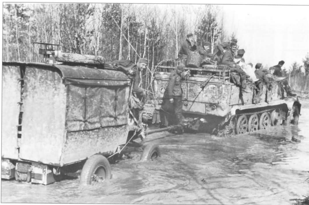
A very shabby Sd.Kfz. 7 tows an equally rickety lorry across a river. It is using a tow bar to conduct the operation, while all crewmen do their best to stay dry. The loaded weight of this vehicle was 11.55-tons, its length 22.6-feet, its width 7.91-feet and its height 8.65-feet.
