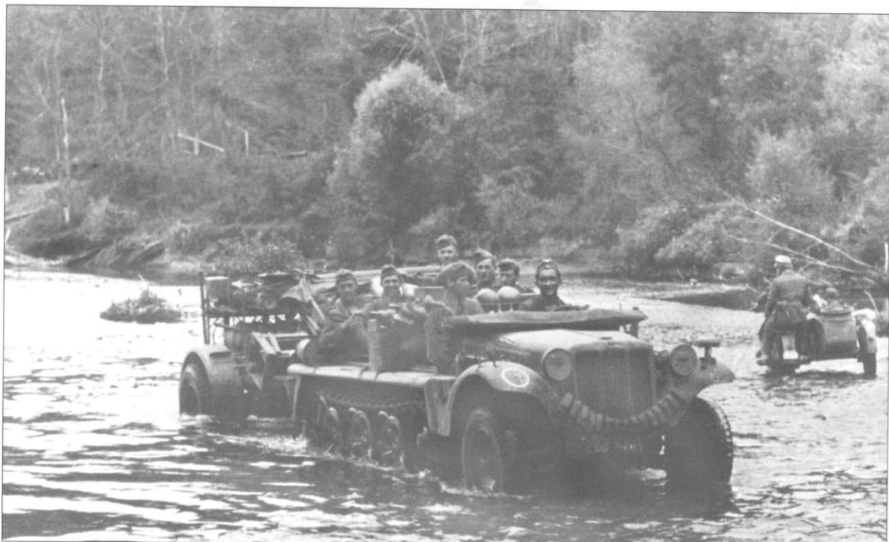
This Sd.Kfz. 10 pulls a trailer consisting of a launcher for 28cm or 32cm Wurfrahmen un-guided rockets, across a river. Note a rocket in its crate, lying across the trailer, as well as the circular unit marking on the front fender of the tractor. The "necklace"-like item hanging in front of the radiator is a string of spare rubber track pads.
